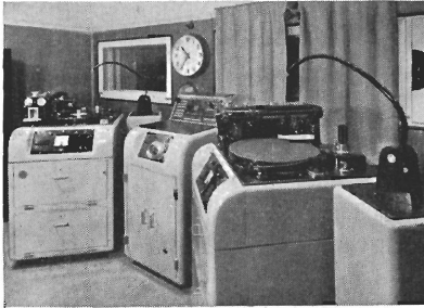
FIG. 61—B.B.C. Disc recording channel, comprising two recording machines, control desk and two suction units for pneumatic removal of swarf.
